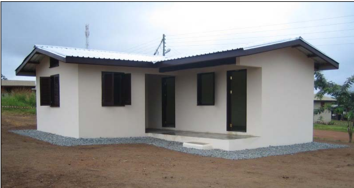
Figure 7.4: Typical Resettlement House
