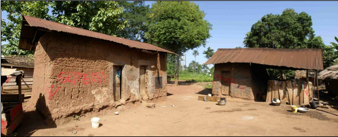
Figure 3.9: Traditional Homestead at Subika
